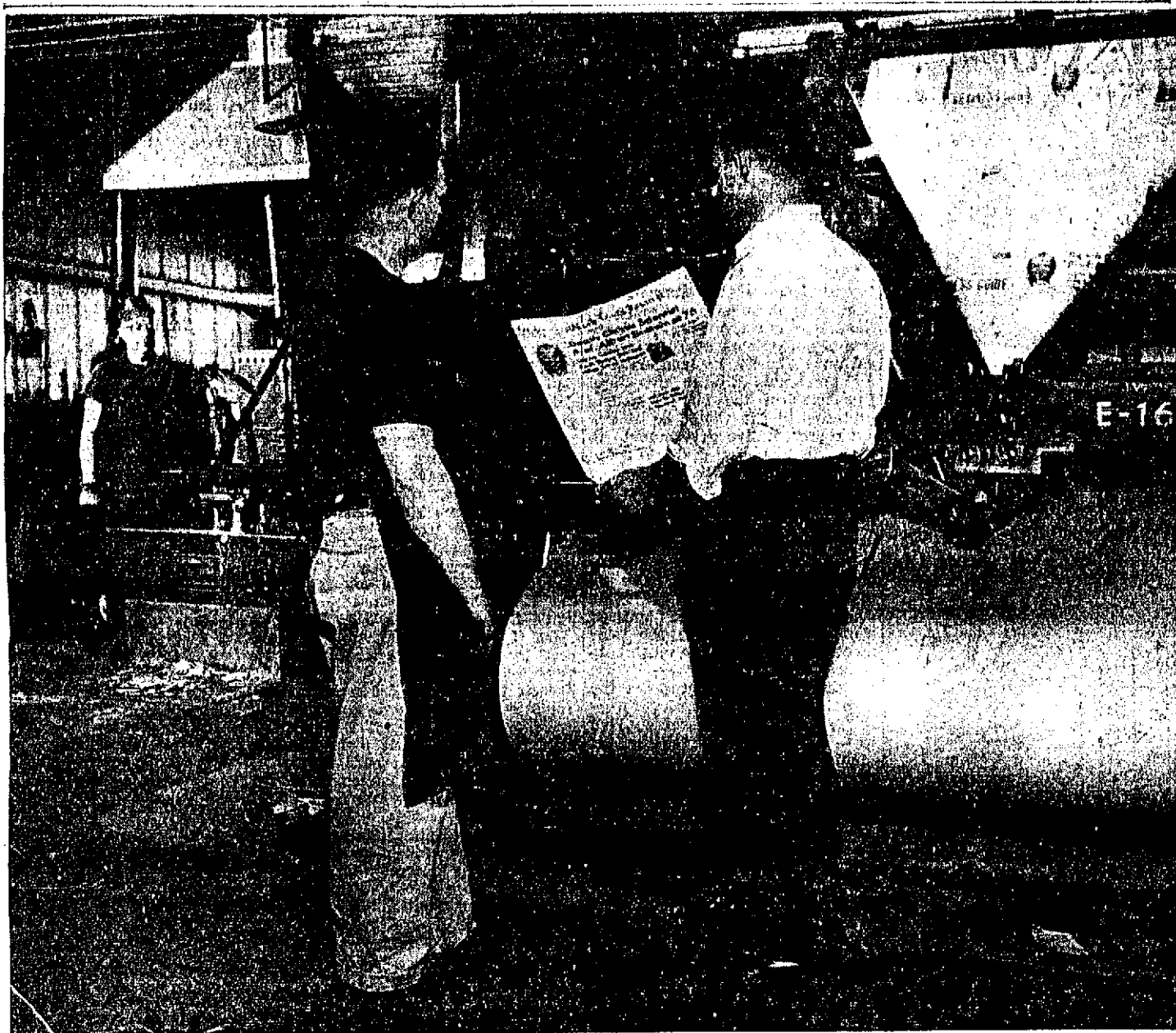
ADDITIONAL PRINTING CAPACITY was provided after conversion to daily by this efficient Goss Duplex 8-page web press. In the foreground (left) Pressman Harold Orr checks the impression on the first press proofs with Mechanical Superintendent Ben Foster (right). At the left in the background is the Journal's stereotyper, L. J. Michaelson, whose job is to make metal castings of the illus-
